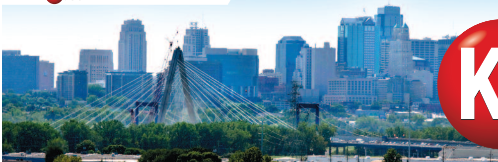
The new Christopher S. Bond Bridge at I-29/I-35 across the Missouri River, will open this October.
